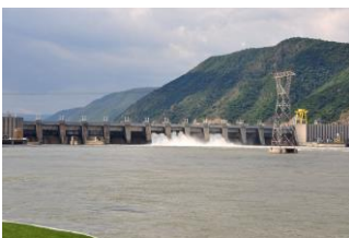
Dam of the Iron Gates - Serbia - Rumania
